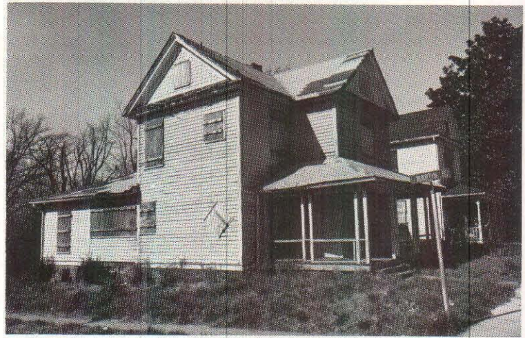
Acquisition of dilapidated housing structures (left) and an active housing rehabilitation program (right) are key ingredients of the Asheboro neighborhood revitalization program.
