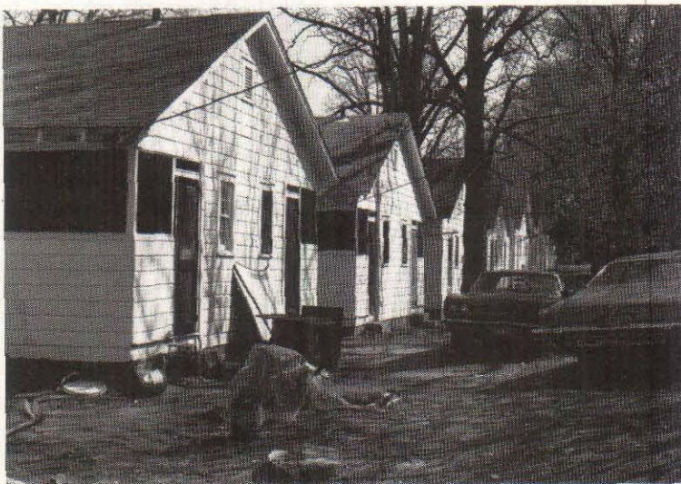
Rear yards of Reid Street development.
