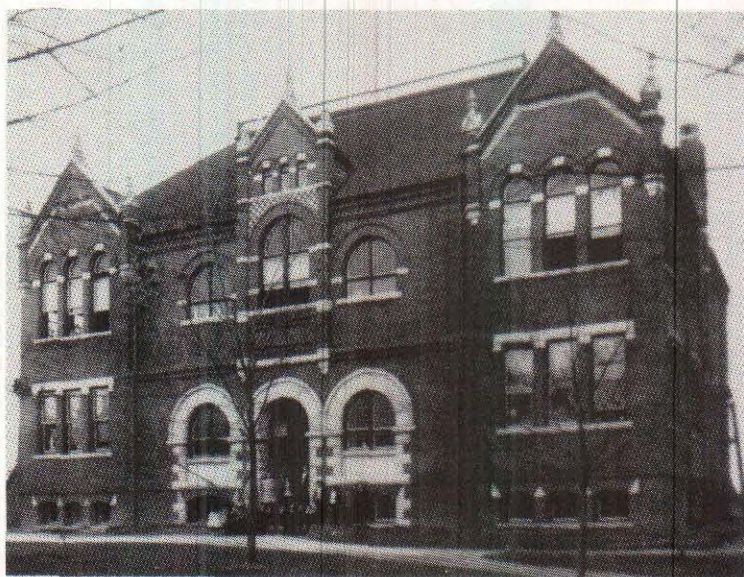
Asheboro Street Graded School. Photograph date unknown.
