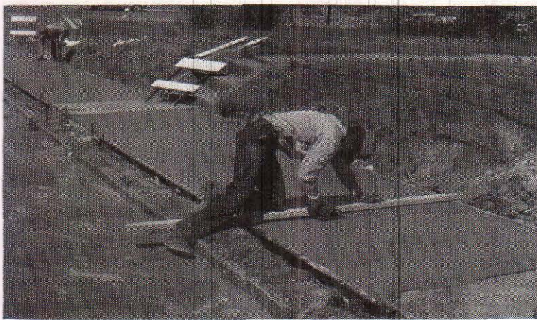
Community Development funded sidewalk improvements underway in the neighborhood.
